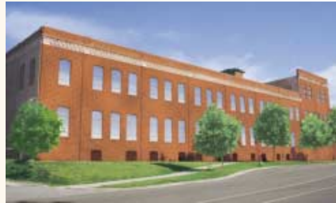
Future rental lofts in New Amsterdam at 6200 Second Avenue (Amsterdam and Second.) Construction begins in Spring of 2001.
